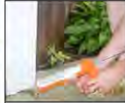
Seal holes on exterior of your house.
